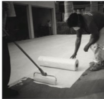
Roll the fabric into the wet Elastomeric a few feet at a time.
