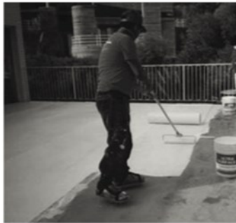
Apply Elastomeric ahead of reinforcement fabric at a rate of 100 sq.ft. per gallon
