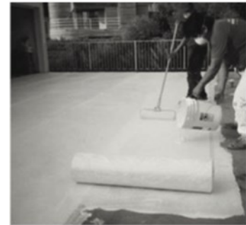
Apply Elastomeric on top of the fabric at 100 sq.ft. per gallon after rolling several feet and lightly broadcast #60 silica sand over top.
