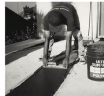
If applying a thin coating system over fabric, it is necessary to first patch the seams with Pro-Surfacer using a trowel or squeegee. Then Apply Pro-Surfacer over entire surface to blend.
